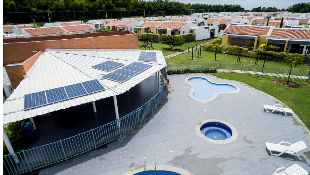
Use of photovoltaic energy for lighting common areas
