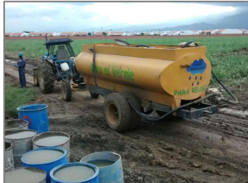
Use of rain water for concrete preparation and cleaning purposes
